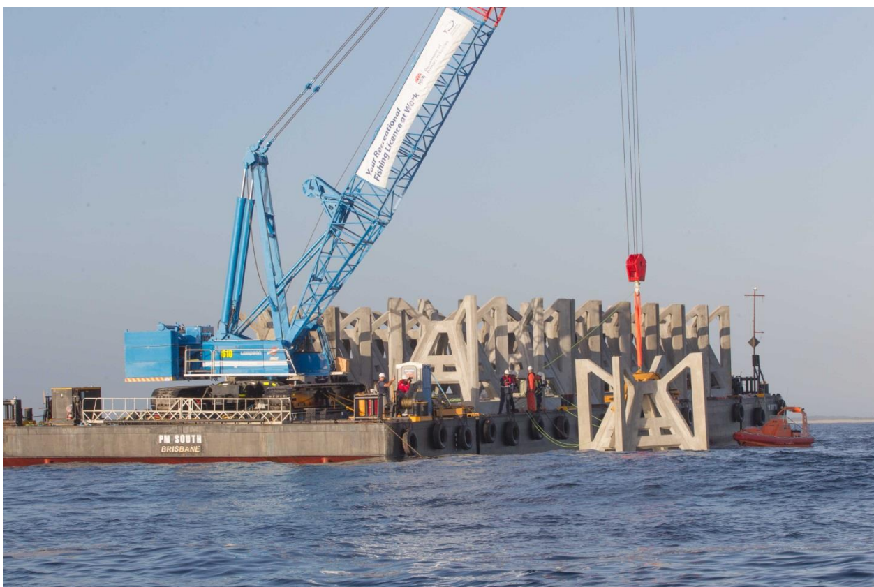
Figure 6. The ReefTemple™ artificial reef modules being installed off Shoalhaven Heads in January 2015
