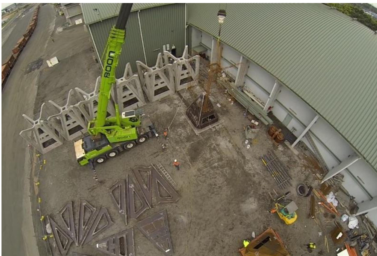
Figure 8. Fabrication ‘hard-stand’ reef module site at Port Kembla in December 2014
