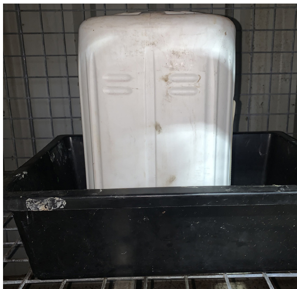
Figure 9. Individual chemical drum bunding can be as simple as a plastic tray.
