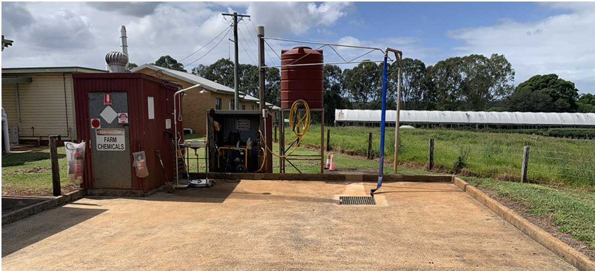
Figure 6. Containment berms are raised structures usually made of concrete that surround the whole storage area.
